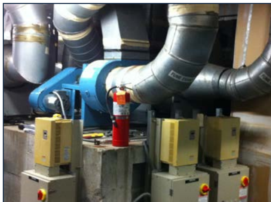
Plenums impeded maintenance (before photo). The TEL solution created redundancy and increased access by combining plenums.
